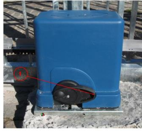
Figure 3: Gate Manual Switch
